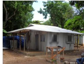
Single family home we wish to build (panel system, unfinished)
